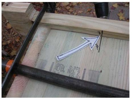
Turn unit upside down and straddle over a saw horse or any narrow projected surface so that the top side base is now resting on a flat surface. Lay the outrigger foot piece as shown flush against the base and align a marked center line on the outrigger foot with a marked center line on the base. Clamp and fasten it to base with six 2½" screws through the predrilled holes.
